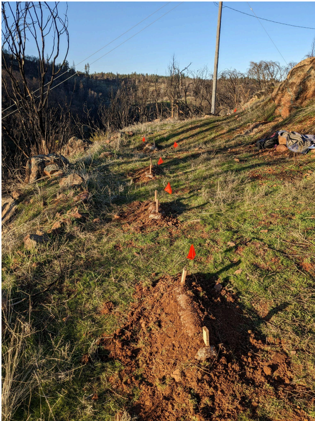
Photos: wattles can be placed on a slope (left), or on flat ground (right); they can be covered with displaced soil (left) or not (right); they can be spread out (left) or aligned end-to-end (right)
