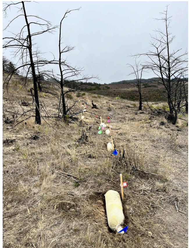
Photos: PFMI wattles deployed around a structure fire (left), and in a burned woodland (right)
