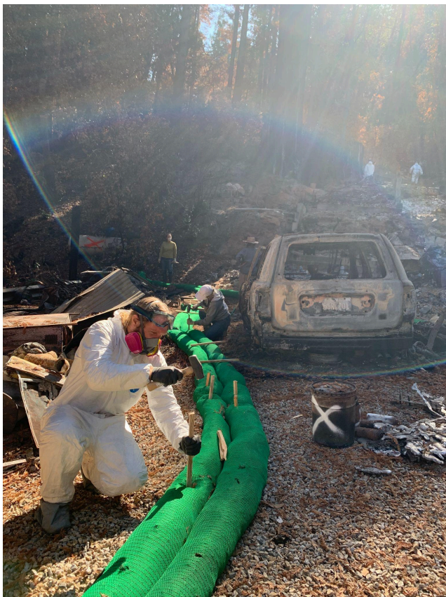
Photos: PFMI wattles deployed around a structure fire (left), and in a burned woodland (right)
